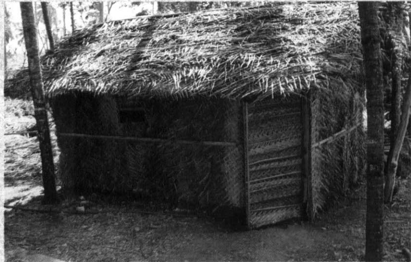
Low cost mushroom house built exclusively of coconut materials
