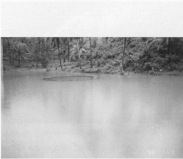
Water harvesting structure to store 50 lakh litres of water
