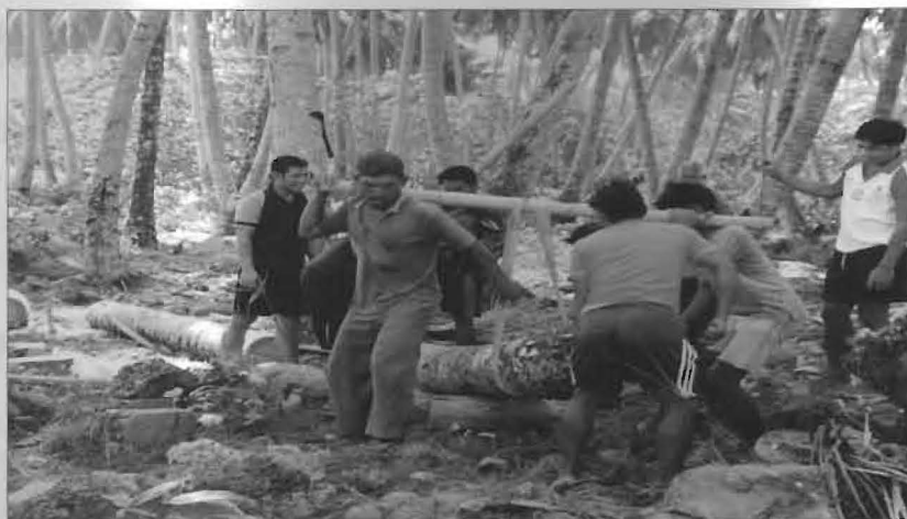
Cutting and removal of old and senile palms
