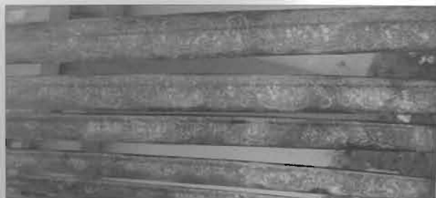
Extensive damage on the lower leaflet
