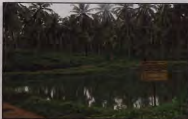
Check dam inside the farm
