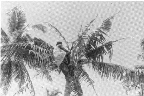
Removal of rotten portion in the crown
