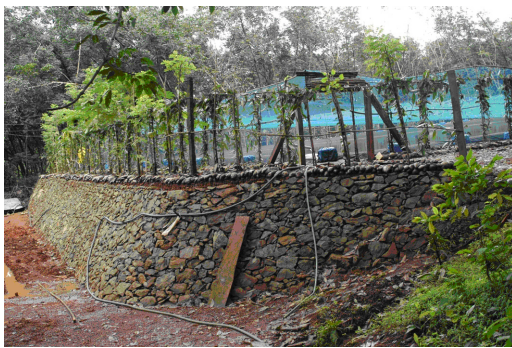
Fig.5. Side of the pond stabilized with rubble pitching
