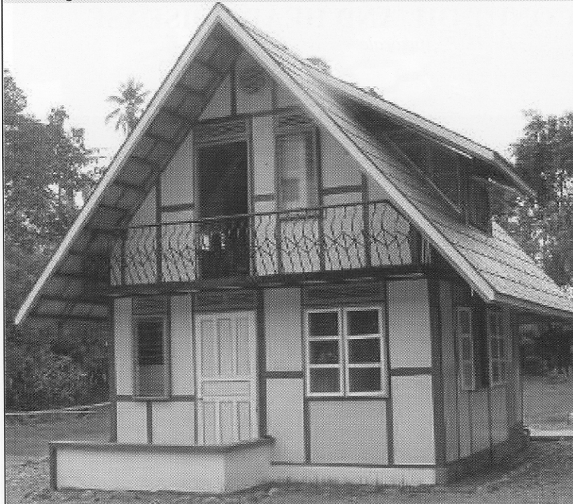
Fig 14. Model house made from coconut wood-coir cement board
