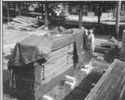
Fig 11. Boron-treated lumber wrapped in plastic cover
